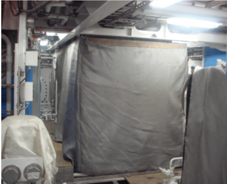
Diesel engine jacking in ships
